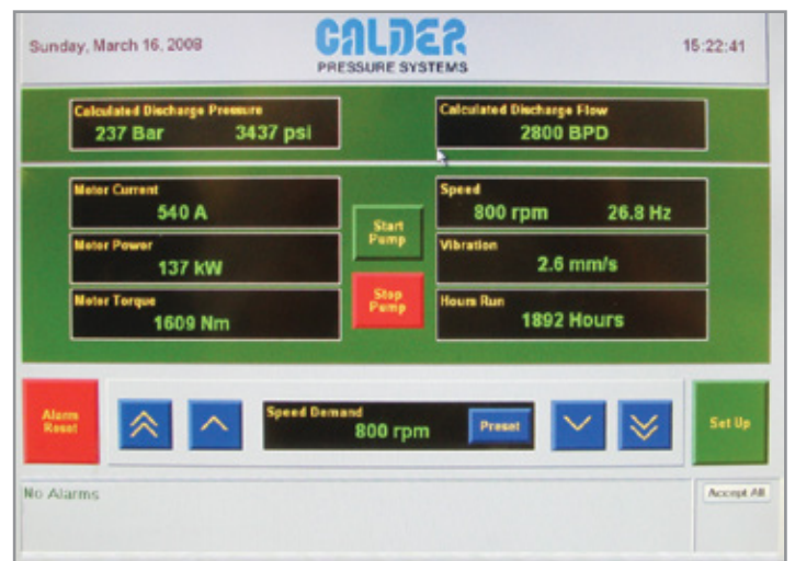
HMI Control Panel.
