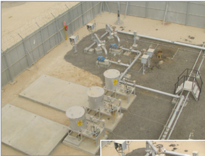
Chemical Dosing & Boost Pumps.
