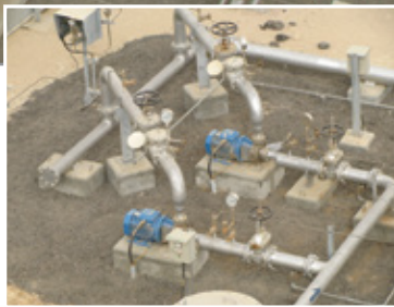
Chemical Dosing & Boost Pumps.
