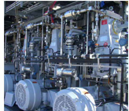
HDP 175 units for methanol duty Op. pressure 5,300 psi – 370 bar Flow rate 46 gpm – 176 l/min
